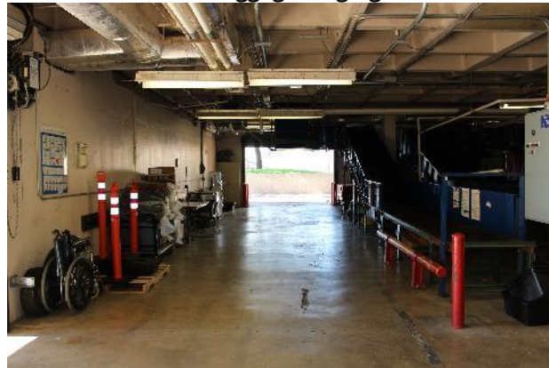
Figure 2-40 Outbound Baggage Staging & Exit
