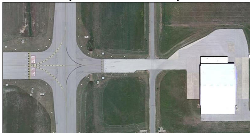
Figure 5-16 Taxiway C1 Intersection with Runway 17R/35L
