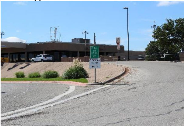
Figure 2-5 Upper & Lower Level Access Roads
