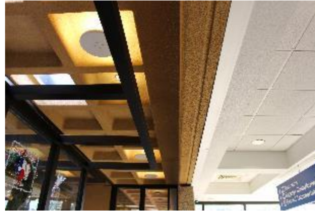
Figure 4-21 Ceiling Change at SSCP
