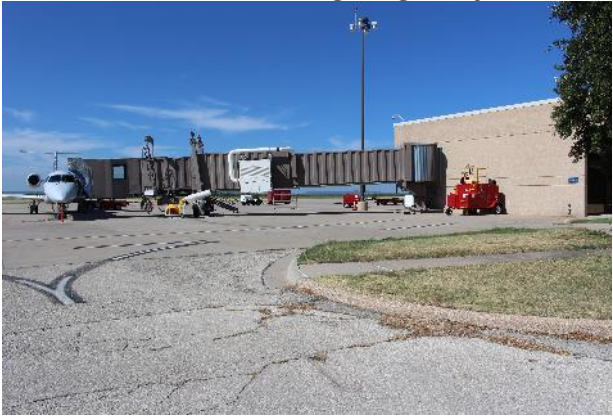
Figure 2-45 PBB at Gate 3 serving a regional jet
