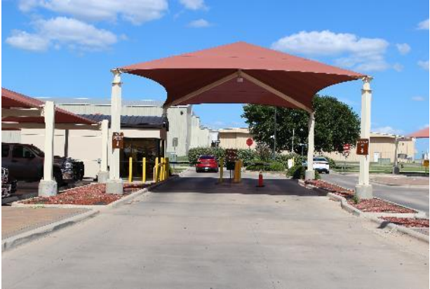
Figure 2-12 Passenger Parking Exit
