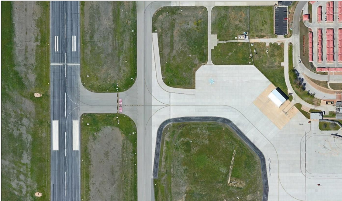
Figure 5-9 Taxiway C1 Intersection with Runway 17R/35L
