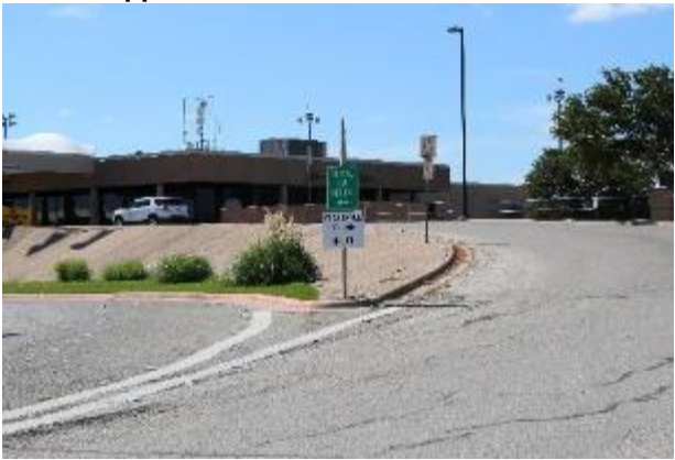
Figure 4-13 Upper & Lower Level Access Roads
