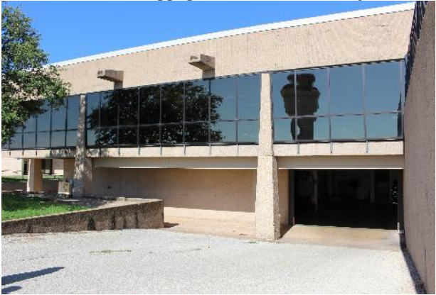
Figure 2-41 Inbound Baggage Entrance Roadway
