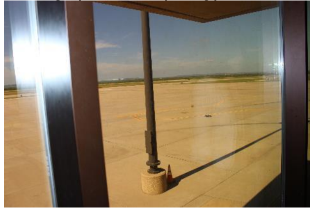
Figure 2-46 Light pole at Gate 1 parking position
