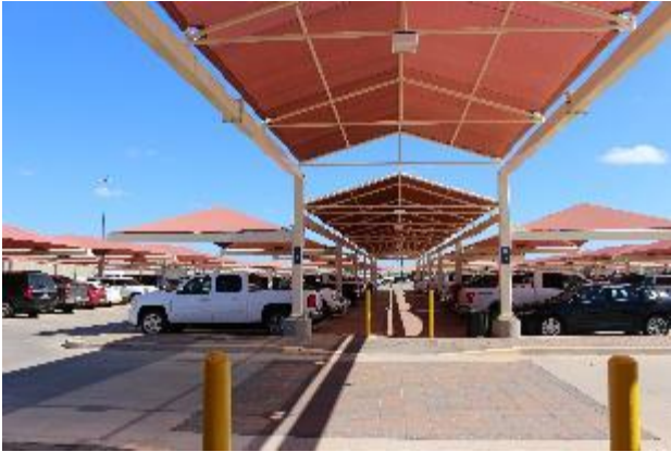
Figure 4-23 Red Concrete Pavers Marking Path Towards Parking
